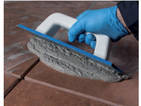
Placing Mapetex Sel N on the first coat of Mapelastich Turbo while till wet
