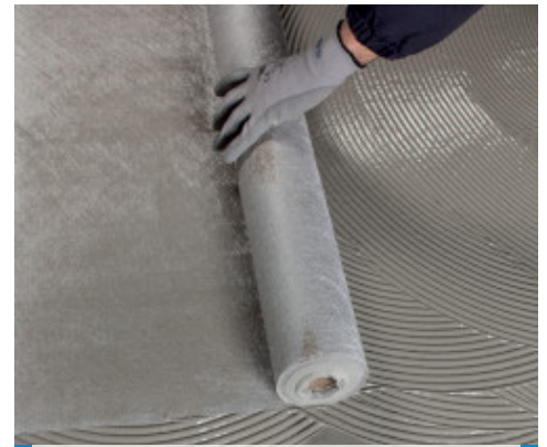
Placing Mapetex Sel N on the first coat of Mapelastich Turbo while till wet
