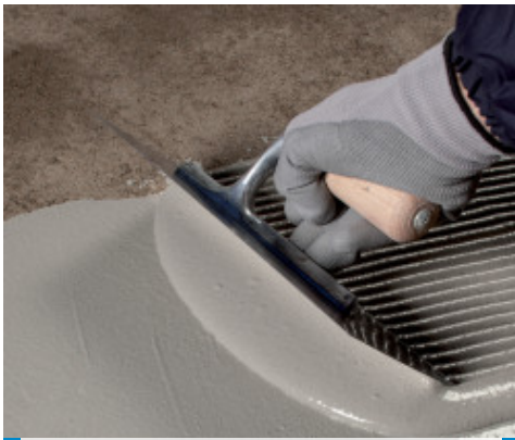
Application of the first coat of Mapelastich Turbo
