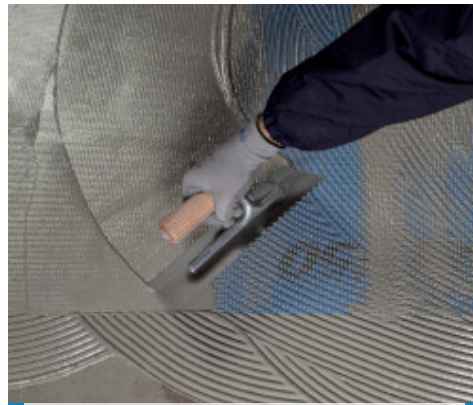
Placing Mapenet 150 on the first coat of Mapelastich Turbo while till wet
