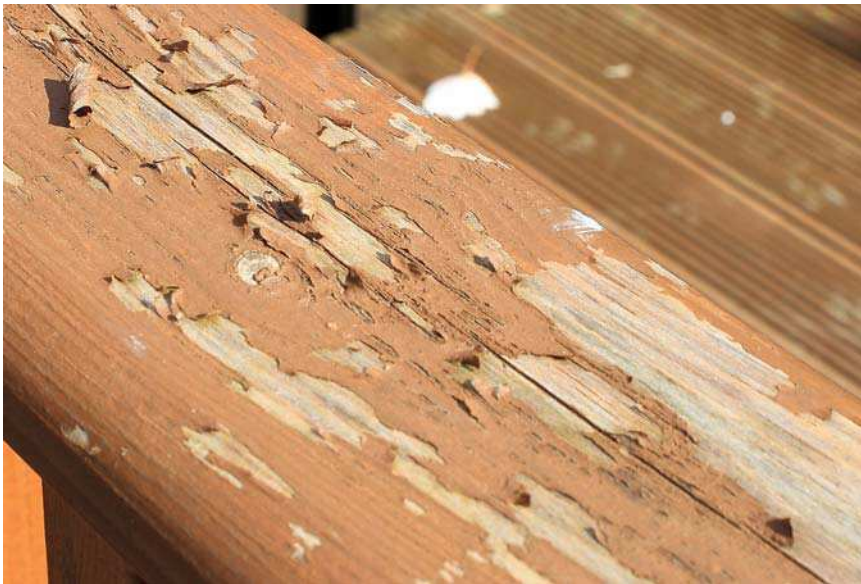
Above shows the detail on a portion of handrail
