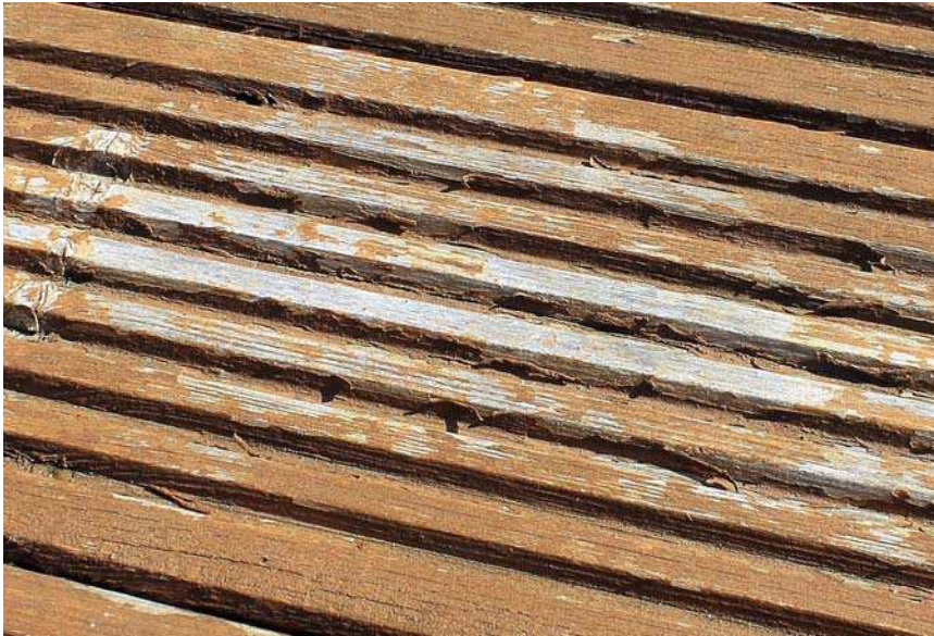
Above shows the detail on decking planks
